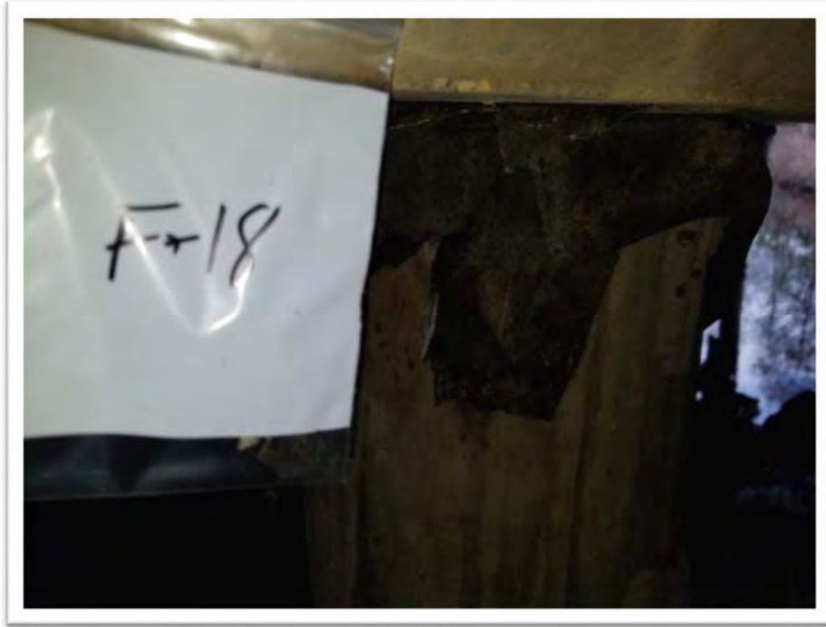
Photograph #25 Sample F-18 – Felt Paper Sampling Point Located Between Wood Piers and Concrete Beams on Bridge 3 (None Detected)
