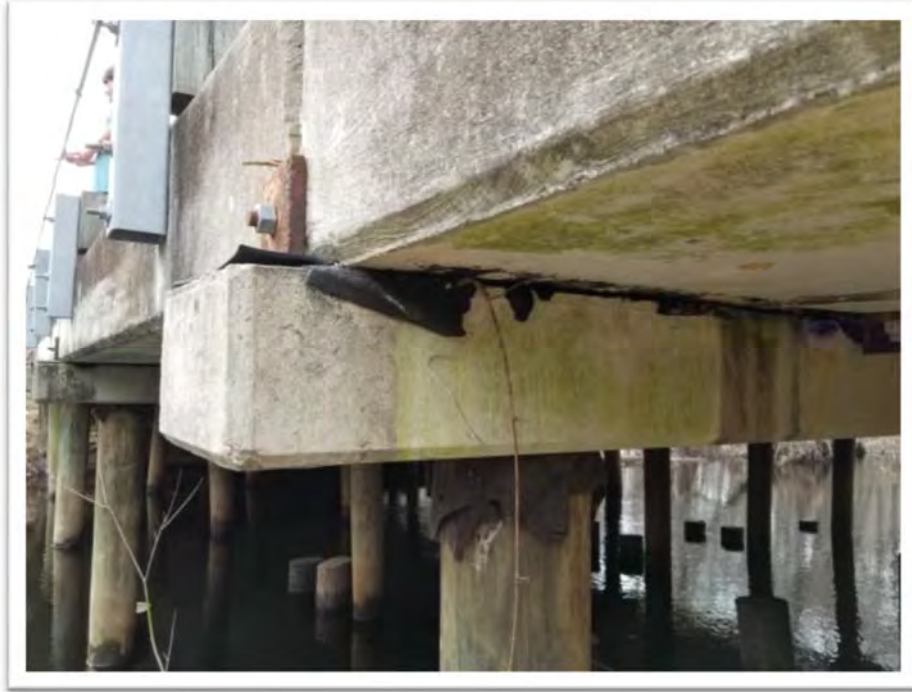
Photograph #03 View of Underside of Bridge 2 – Looking Northwest
