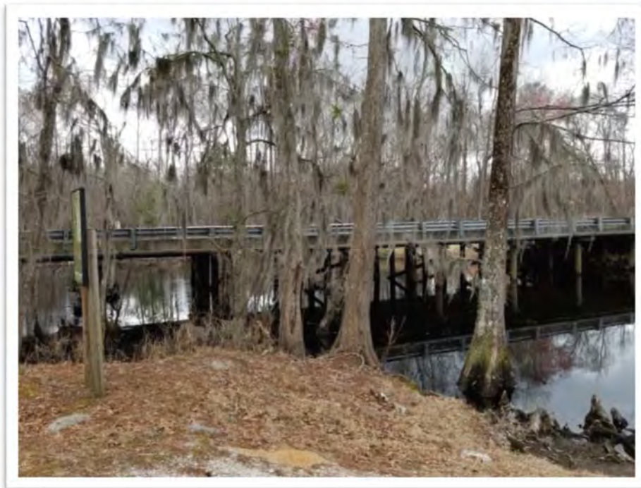
Photograph #16 Bridge 3, Structure No. 1770004500300 – Looking Southeast
