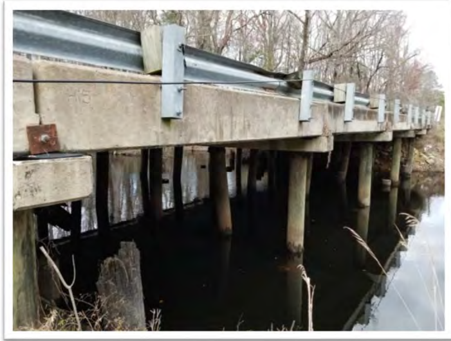
Photograph #05 Additional View of Bridge 2 – Looking Northeast
