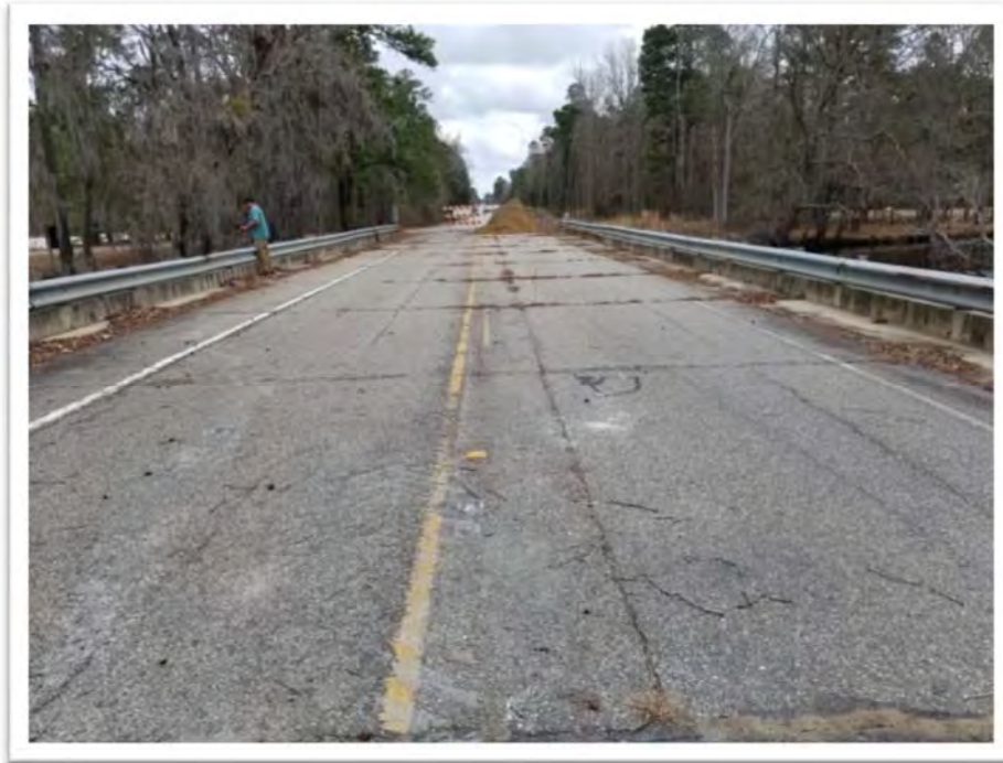
Photograph #15 Bridge 3, Structure No. 1770004500300 – Looking Northeast
