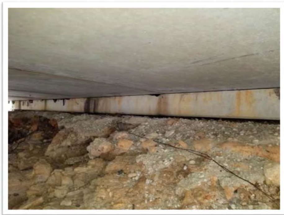
Photograph #06 Bridge 2 Abutment – Northeast End of Bridge
