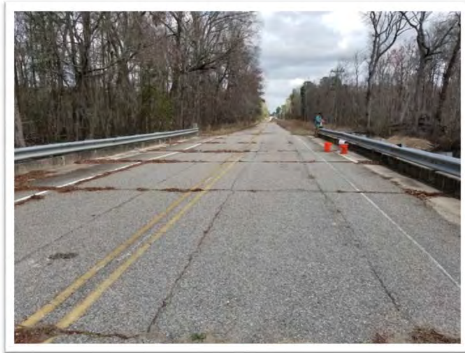
Photograph #01 View of Bridge 2 – Structure No. 1770004500200 – Looking Northeast
